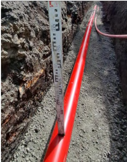
Plate 4-11 Typical Single Cable Trench View
