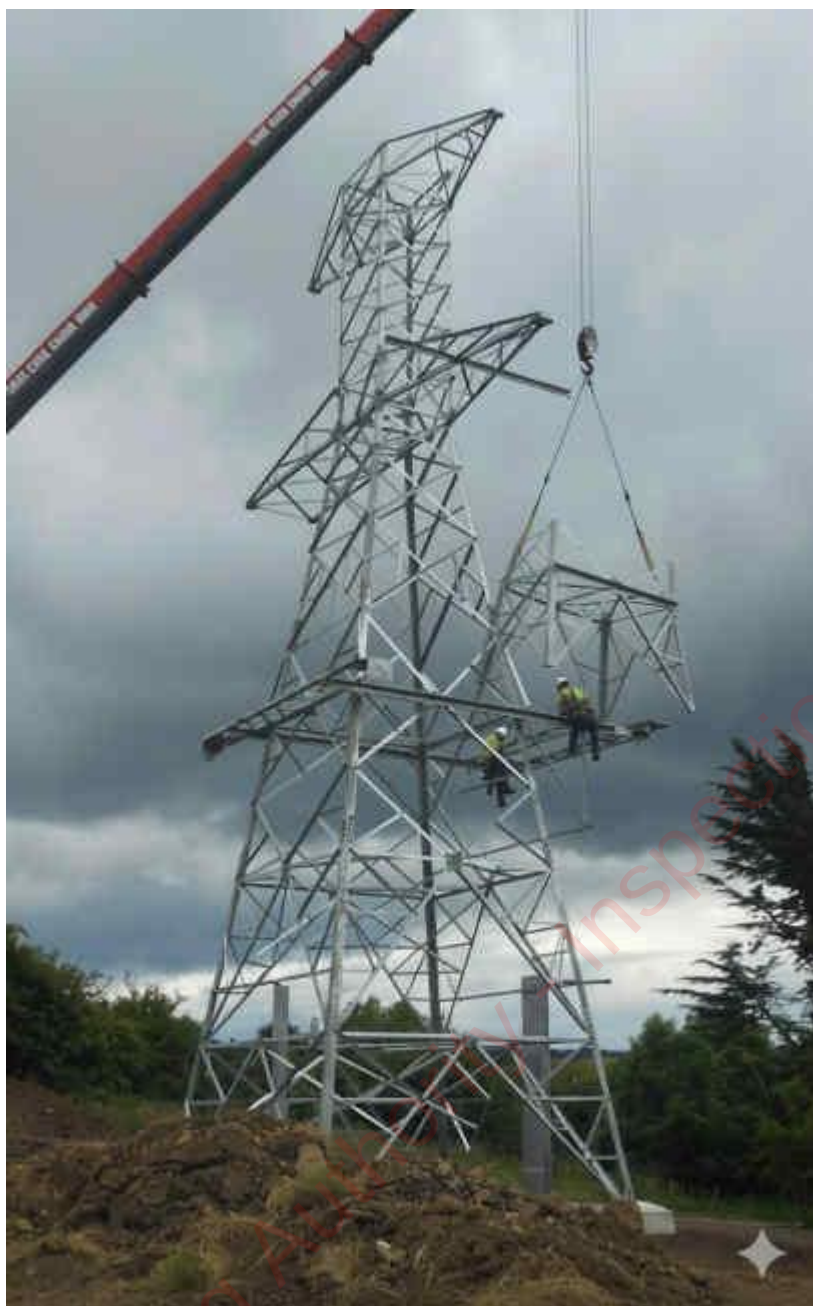
Plate 4-21 End Mast under construction
