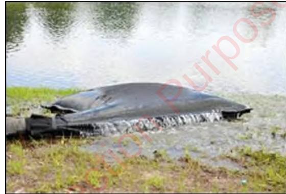
Plate 4-8 Silt bag under inspection
