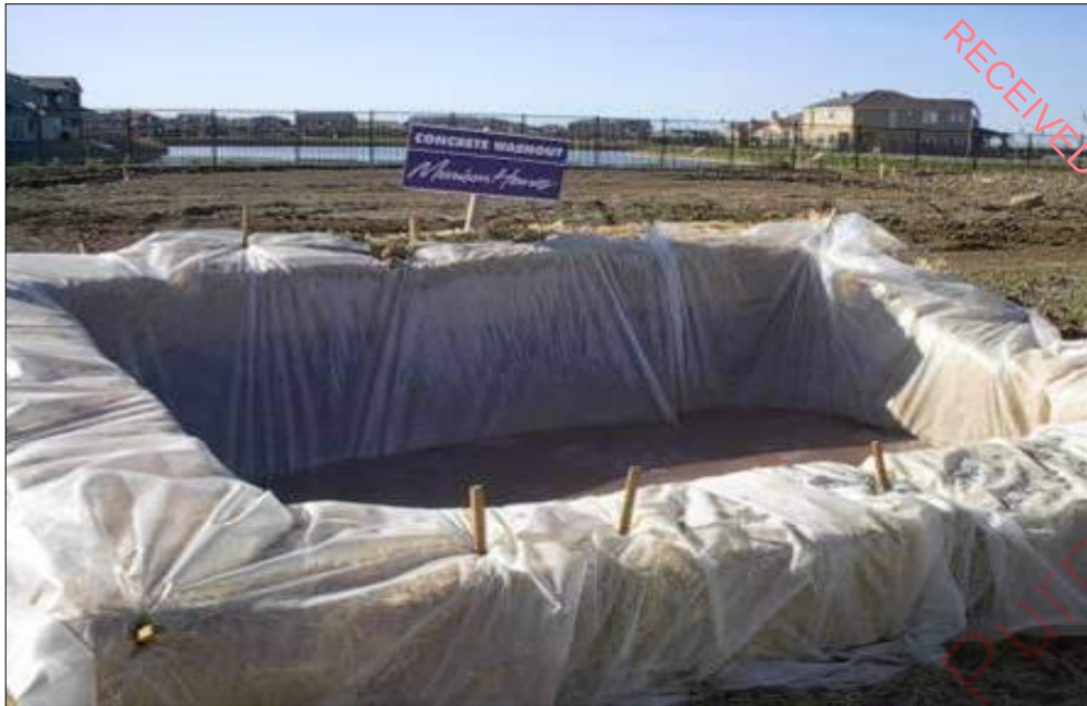
Plate 4-4 Concrete washout area
