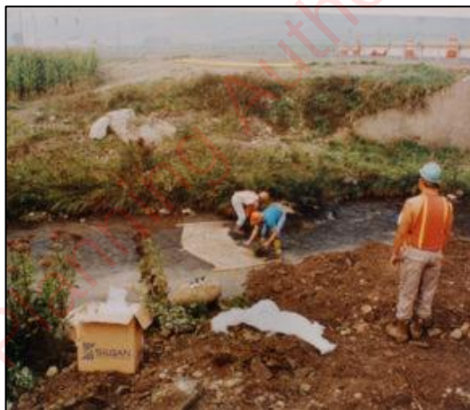
Plate 4-9 Typical Sedimat Details (Source: https://www.hy-tex.co.uk/ )
