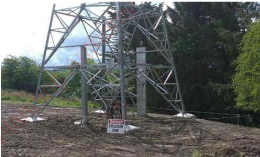
Plate 4-20 Base of end mast structure backfilled
