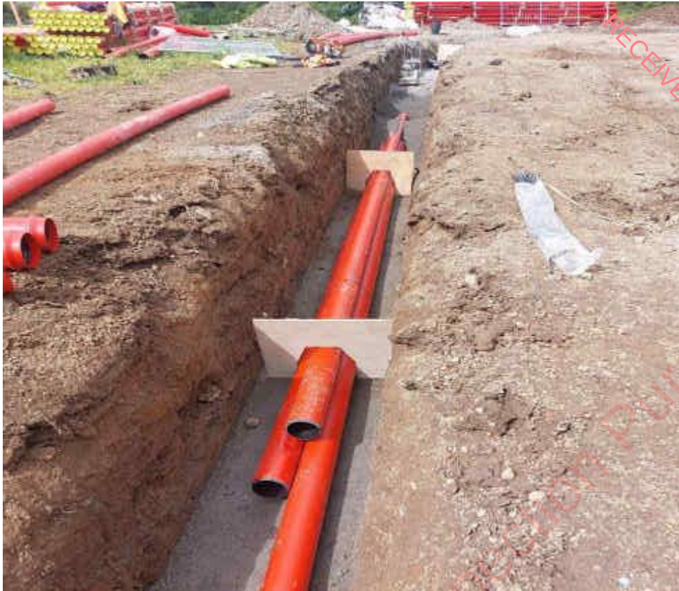
Plate 4-15 Typical 110kV underground duct installation on private land
