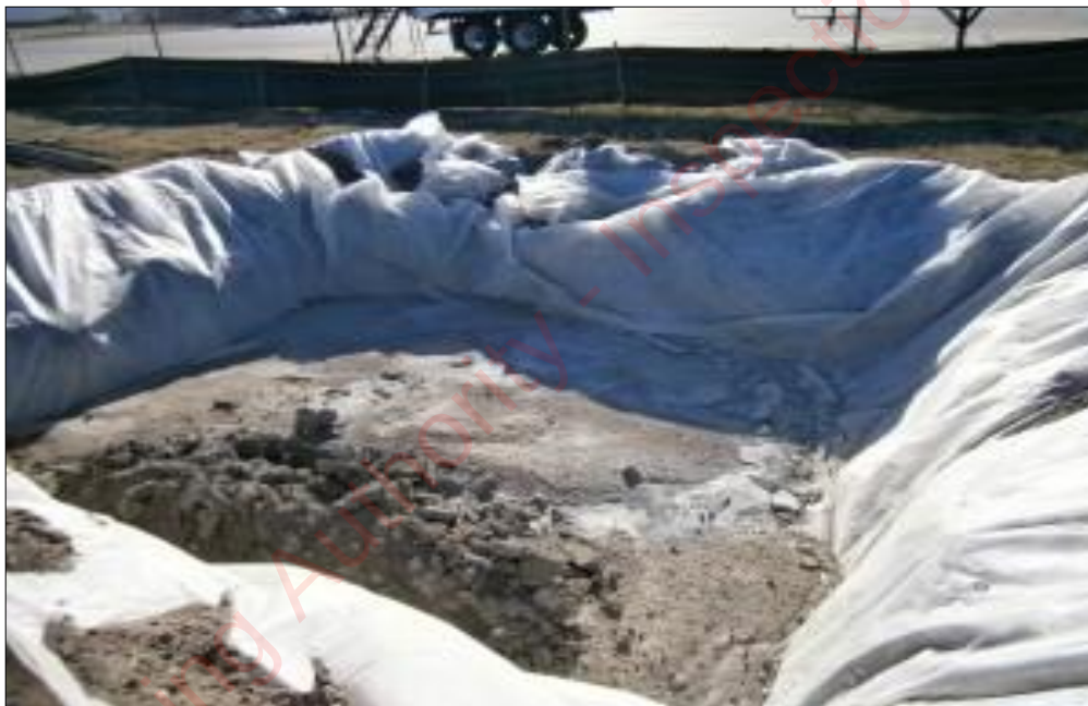
Plate 4-5 Concrete Wash Out Area
