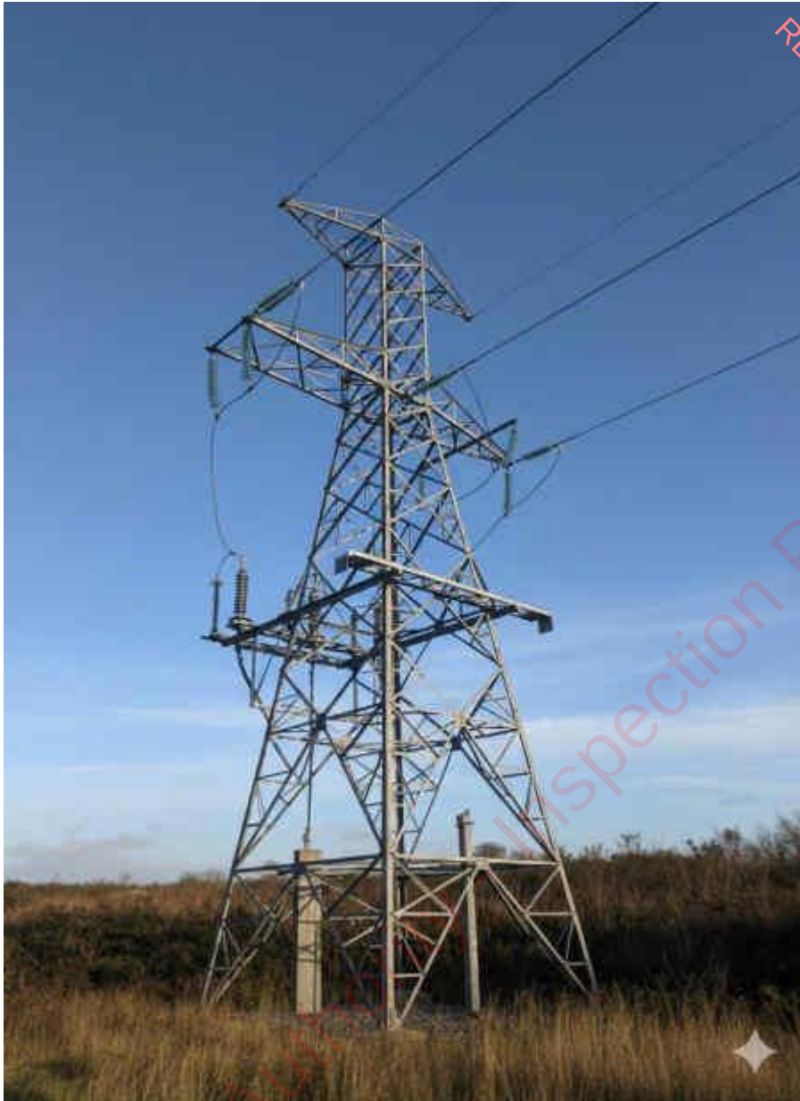
Plate 4-22 Cable end mast
