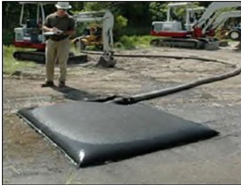
Plate 4-7 Silt Bag with water being pumped through
