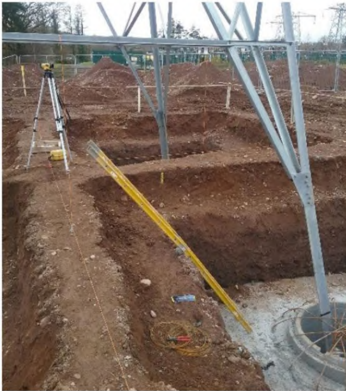
Plate 4-19 Typical 110kV end mast foundation excavation (example image)
